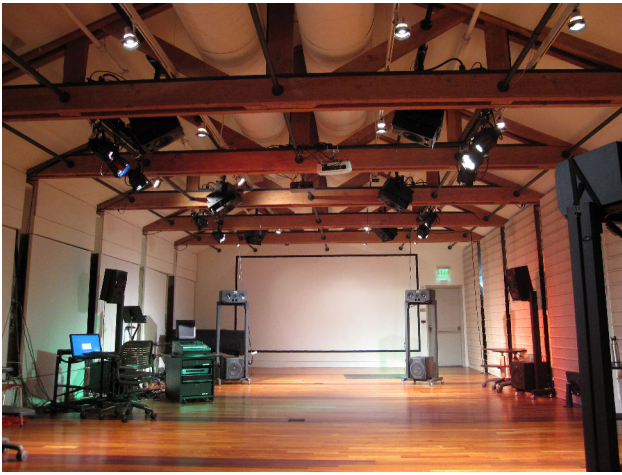
Figure 8. The Stage in 2011, 16 speakers in 8 + 8 configuration, 8 subwoofers in the bottom of the main towers
