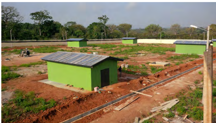
Figure 32 – Construction of New Ammunition Storage Infrastructure in Côte d'Ivoire. 139)
