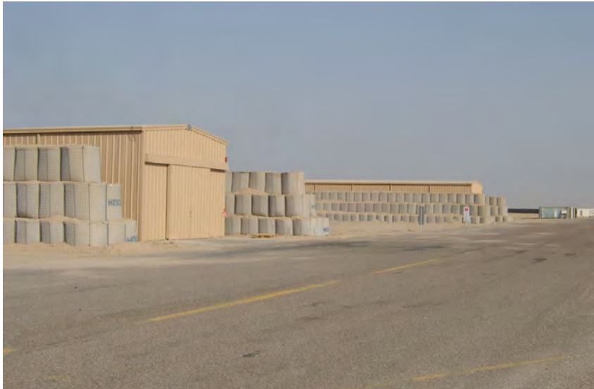
Figure 22 – Barricaded Light Walled Frangible Ammunition Storage Solution. 102)
