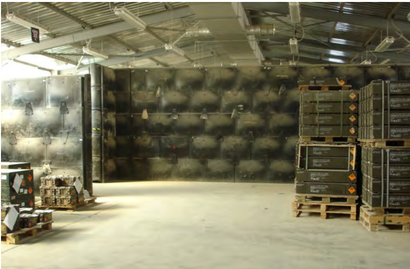
Figure 9 — Water Filled Barriers in a Multi-National Ammunition Storage Point. 61)
