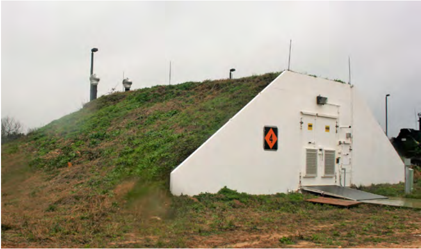
Figure 25 – Pre-Fabricated Metal Earth Covered Magazine - As Built. 105)
