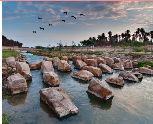
Check dams and Stones features
