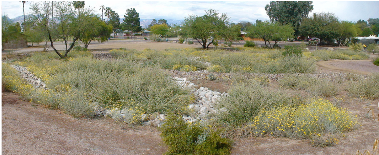
The site is seeded with native plants and featured with check dams to catch and infiltrate water runoff
