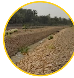
Hanifa valley natural drainage channel
