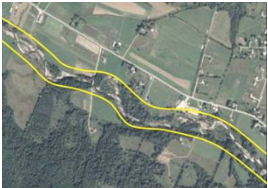
Defining and protecting the meander belt or stream width corridor that will accommodate equilibrium conditions may be the most important objective in any stream restoration and flood recovery project.
