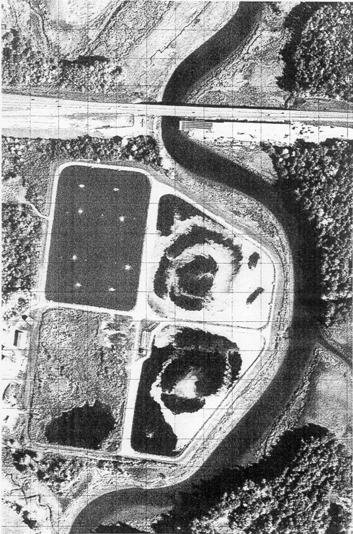
Figure 31. 1995 image of site 8 - Sewage Treatment Plant.
