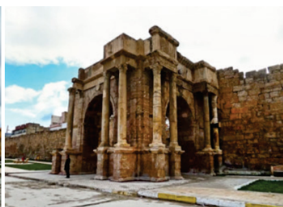
b- North and East spans
