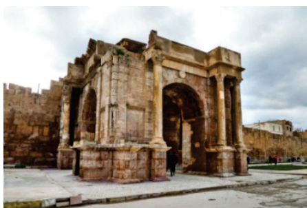
a- North and West spans
