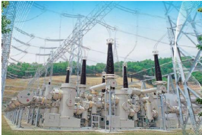
Gambar 2.4. Gardu Induk Gas Insulated Substation (Sumber: BSE Gardu Induk)
