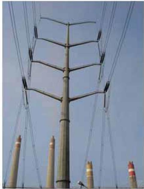
Gambar 4. Tiang saluran tubular steel pole
