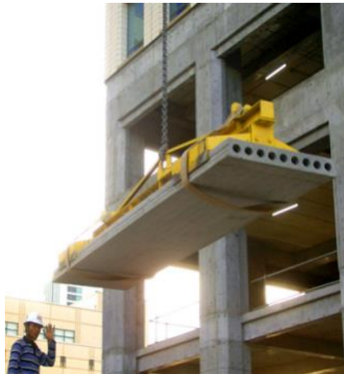
Gambar 3.1. Precast Hollow Core Slab
