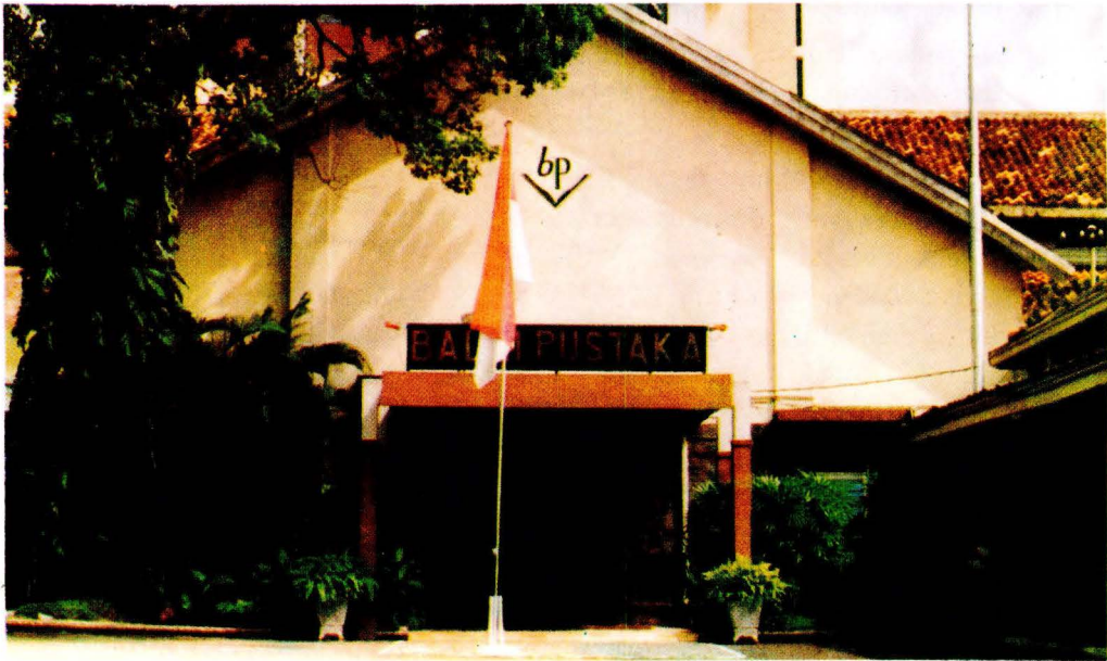
Gedung Balai Pustaka lama The old building
