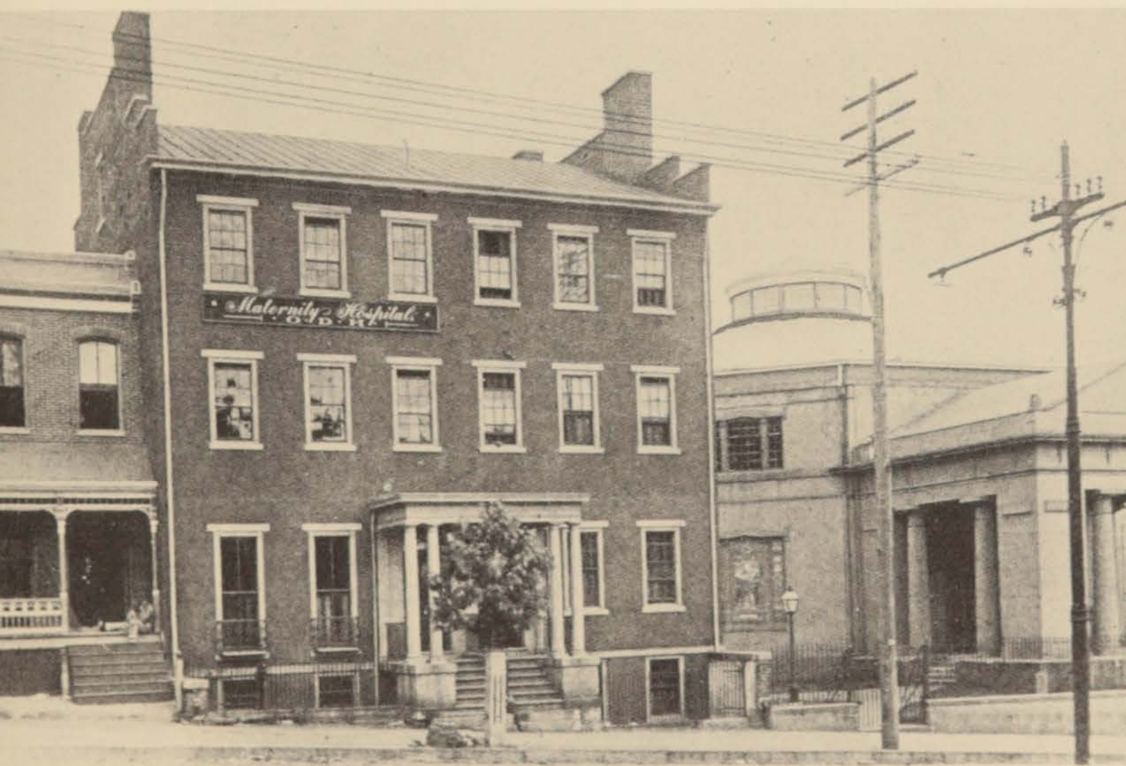
Maternity Hospital Broad Street next to Monumental Episcopal Church.
