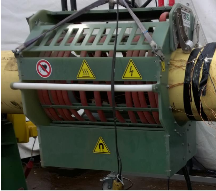
Figure 6: Induction heater installed around field joint.
