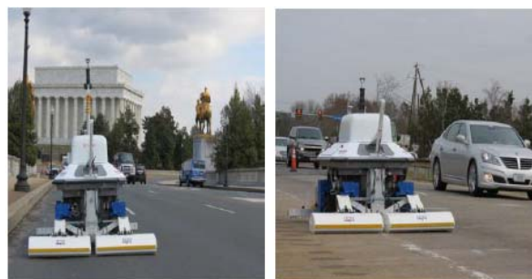
Fig. 3 Operation of GPR bridge deck assessment robot [14]
