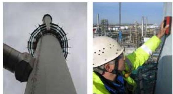
Fig. 1 Manual GPR based NDT on a concrete tower [13]
