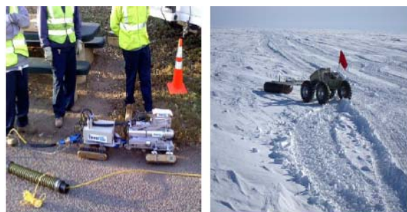
Fig. 4 Sewervue [15] and Yeti Robot [16] in operation
