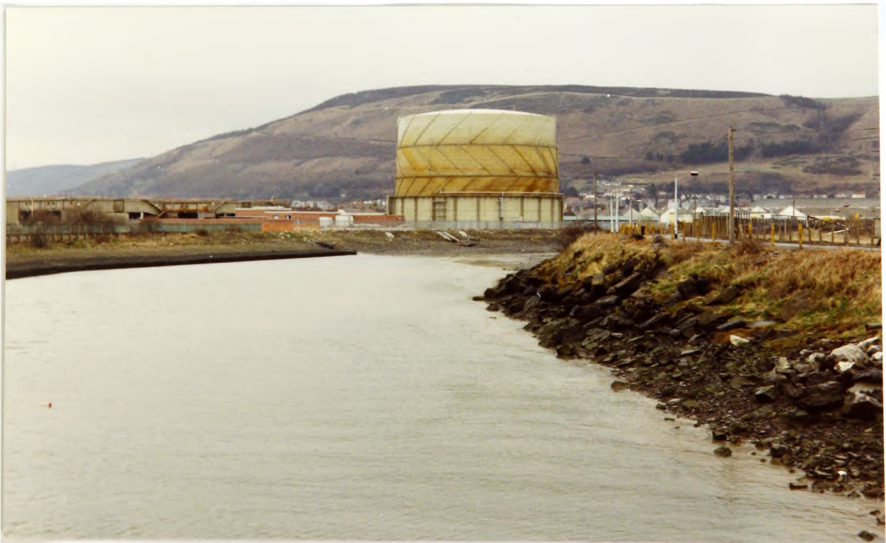
Plate 66 - River Afan Pt 4
