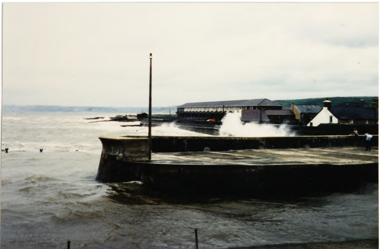
PLATE 4.2 Storm waves breaking over Aberaeron seawall (8.10.83)
