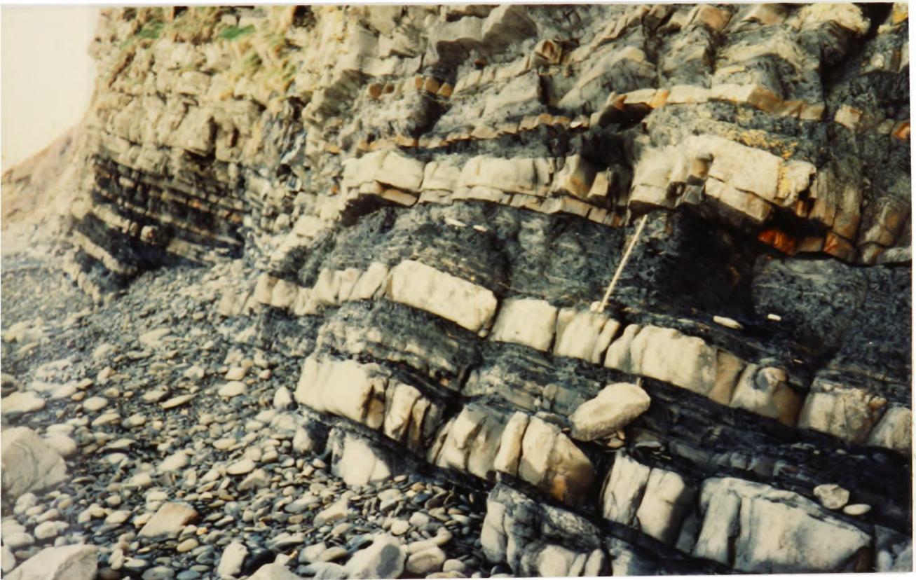
PLATE 9.4 Alternating beds of greywacke and mudstone near Graig Ddu rockfall
