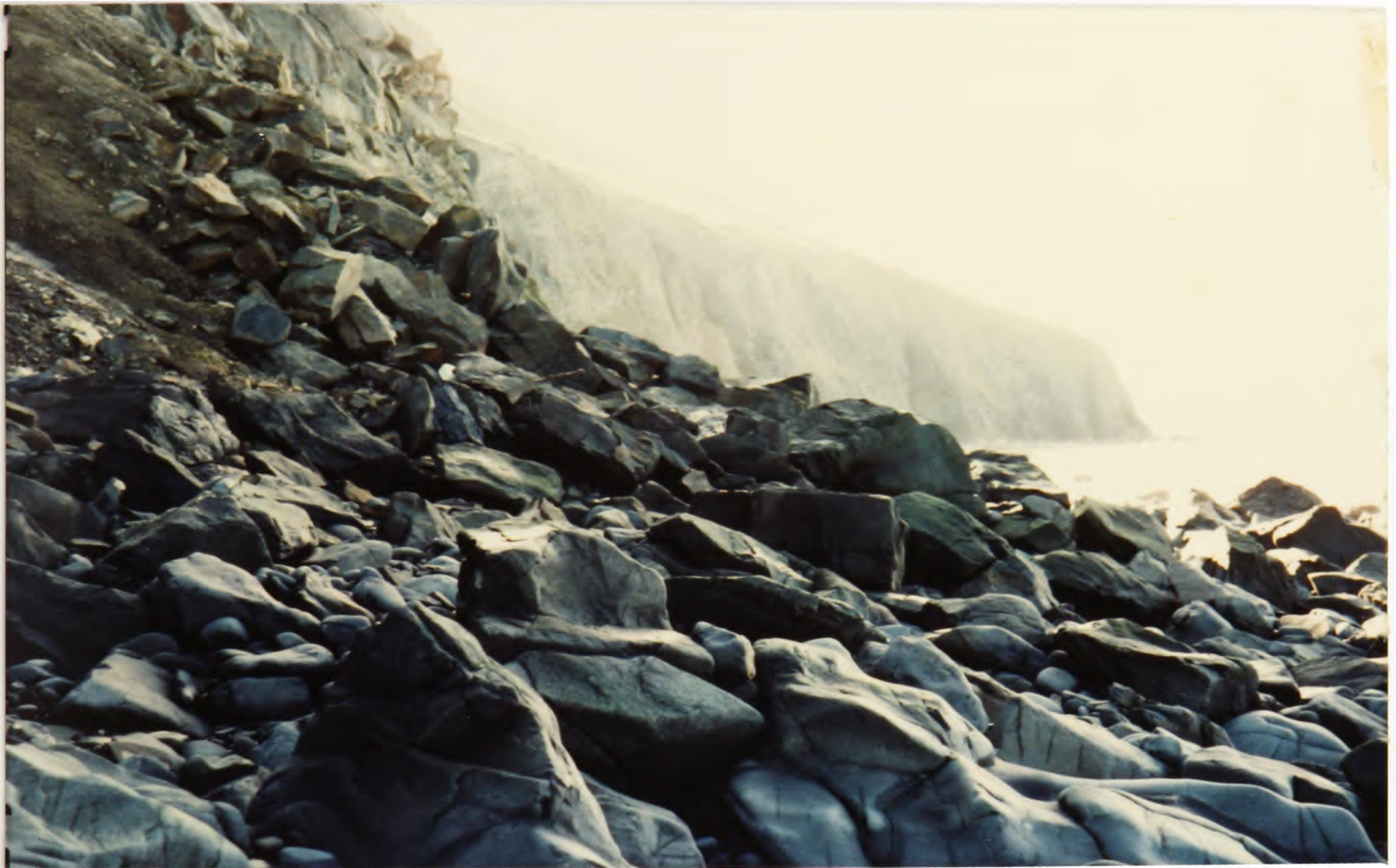
PLATE 9.5 Rockfall near Graig Ddu (Feb 1987)
