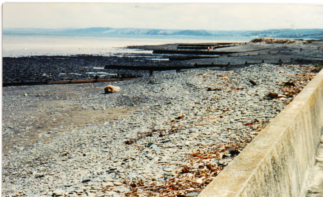
PLATE 3.7 Coastal protection works at Aberaeron north beach
