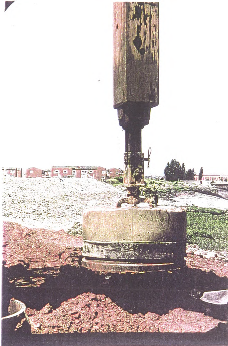
Plate 3.1 A load cell being installed in a test pile hole
