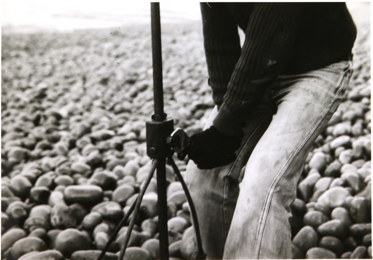
PLATE 26 Fixing the steel collars.
