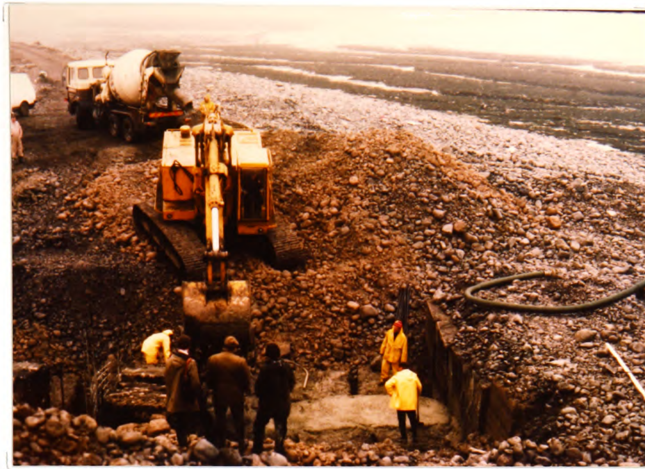
PLATE 3a Welsh Water Authority excavation of Gileston Beach.
