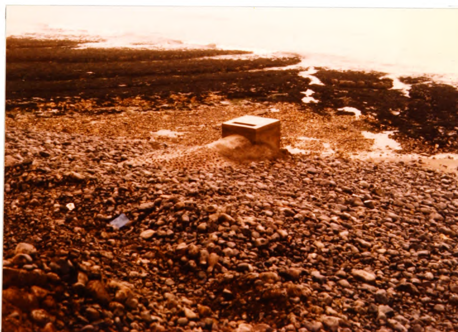
PLATE 3f The seaward outfall.
