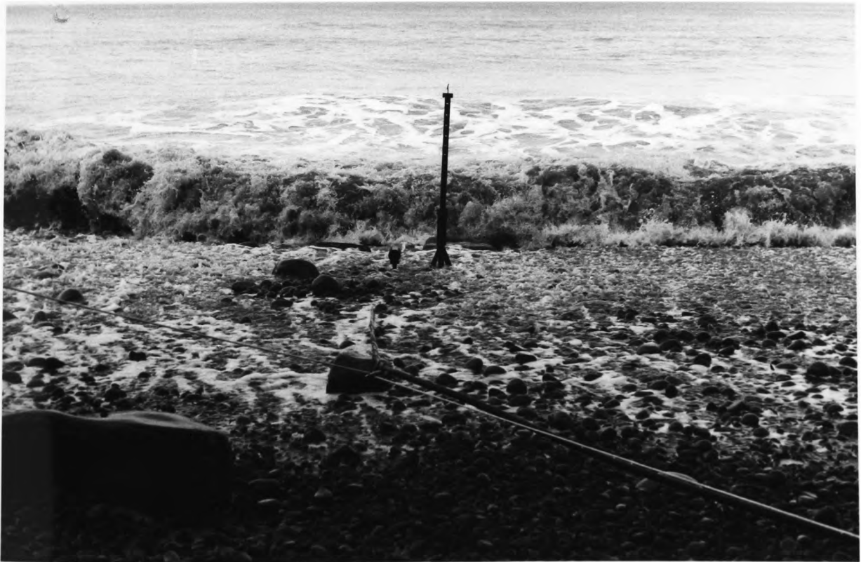
PLATE 32 The transmission cable strapped to hawser and anchor line.
