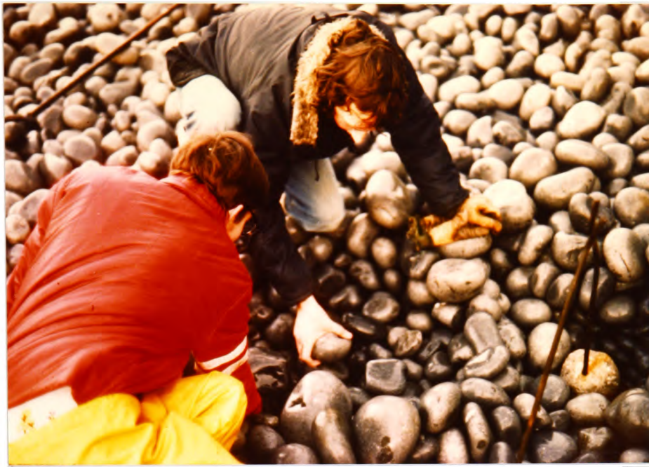
PLATE 25 Burying the concrete support legs.
