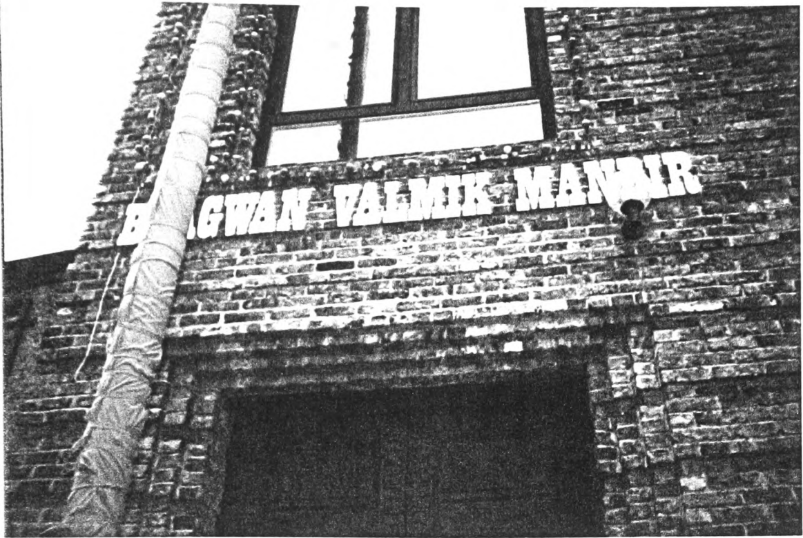
4:11 The sign outside the Southall building, illustrating it as a Vālmīki mandir
