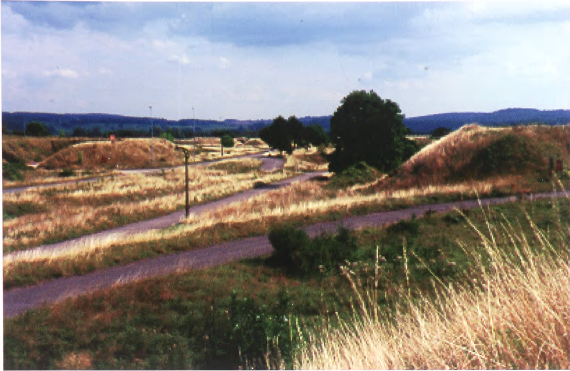
Plate 1.1 General view of revetments at RAF Caerwent.
