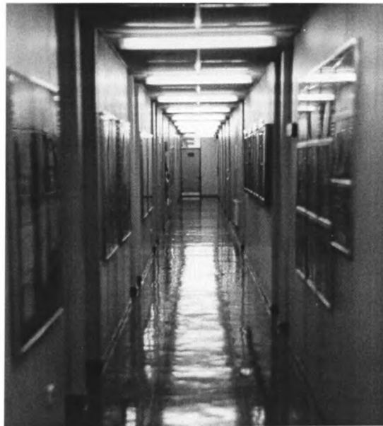
Figure 4-18: Corridor J3, view of wall B
