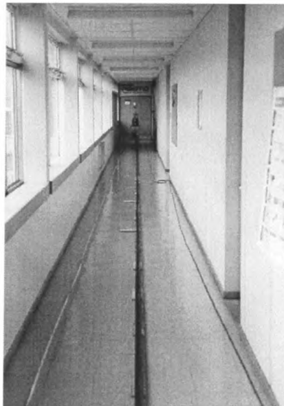
Figure 4-16: Corridor J2, view of wall B
