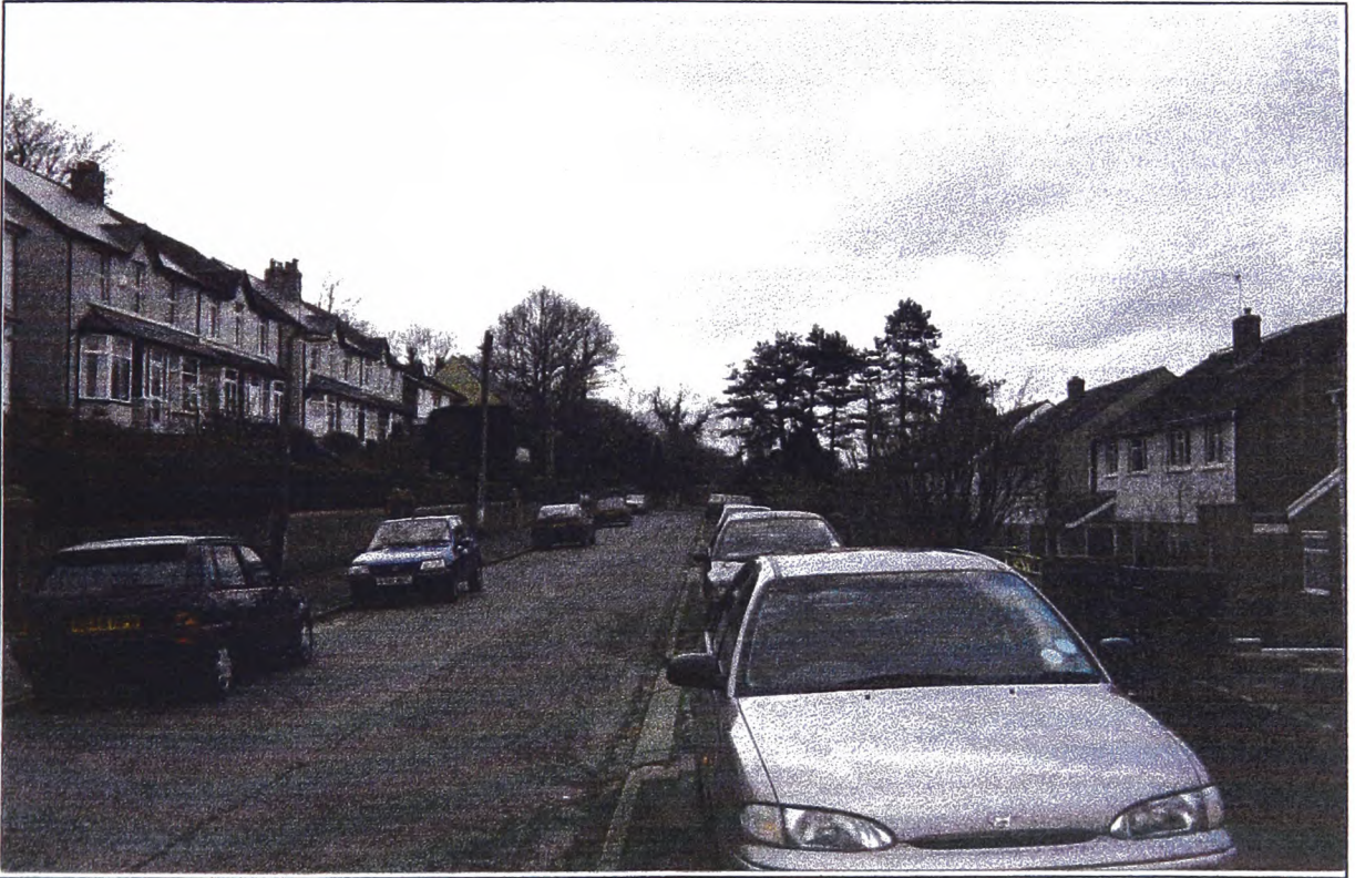
Pencoed Avenue: View looking South
