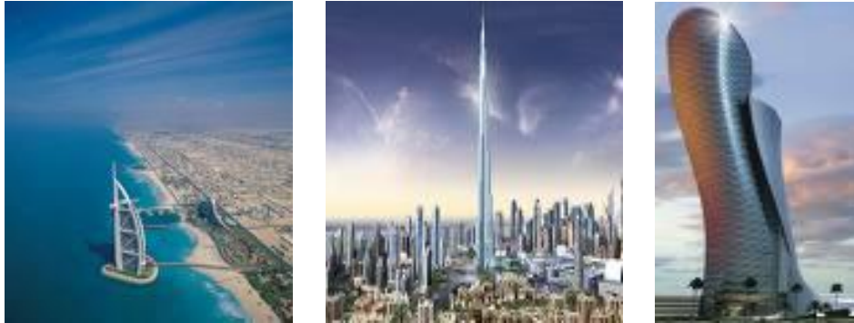
Figure 2.4: Modern Architecture in the UAE
