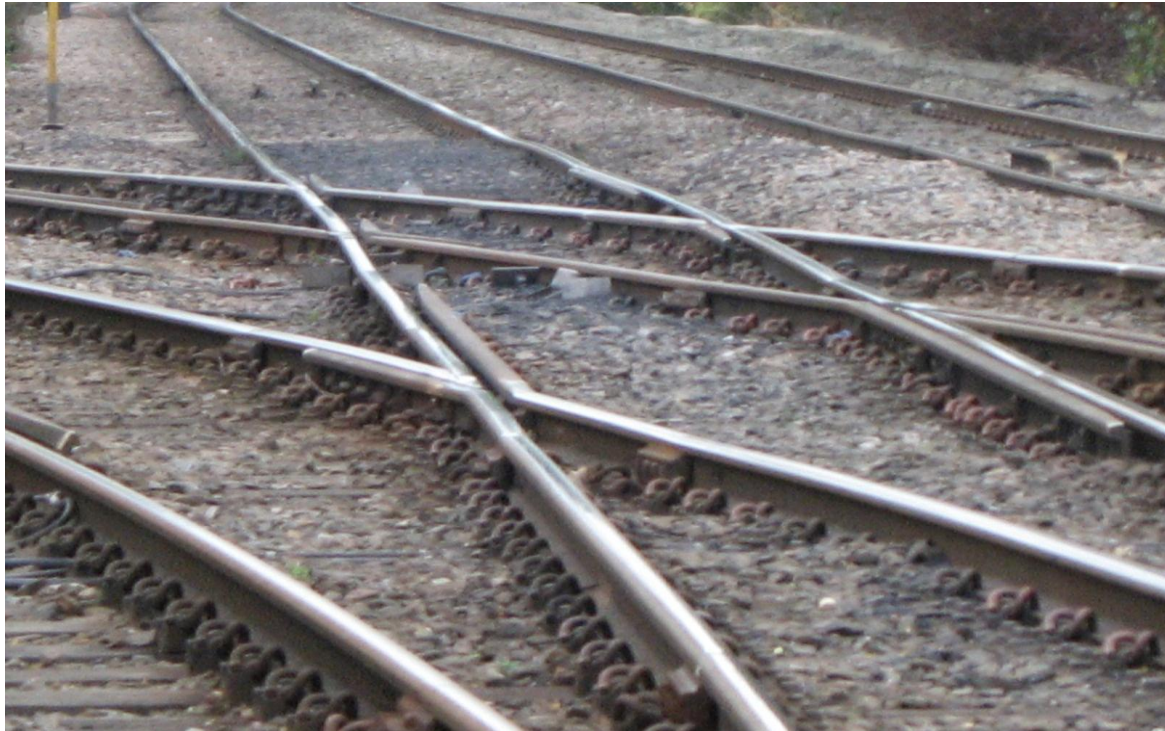
Figure 7: Work in Progress - Early Life Extension Techniques Erewash Valley (source: author)
