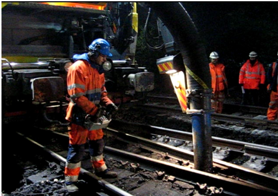
Figure 39: Wrawby Junction; first use of Railvac in a coal spillage area. (Source: author)
