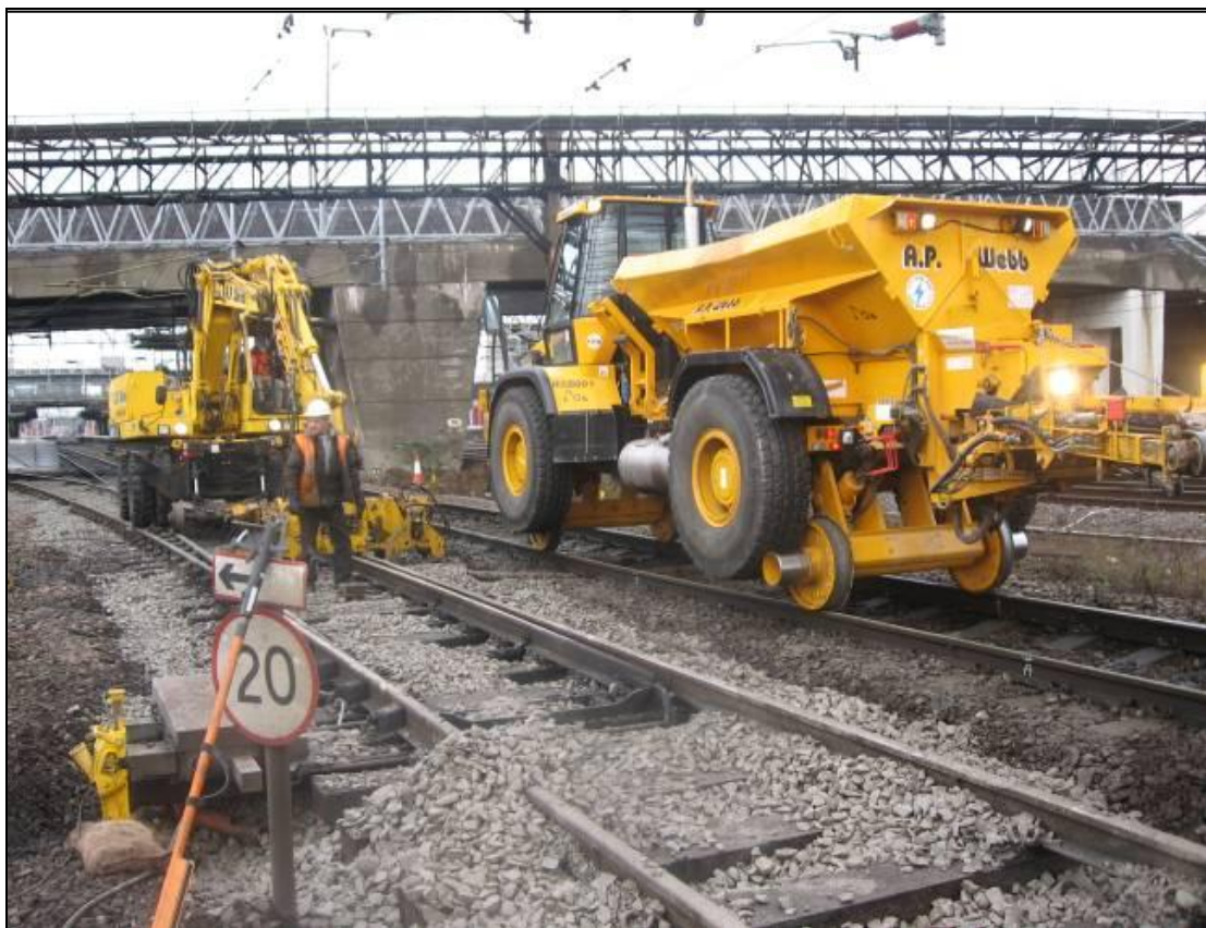
Figure 13: Railvac working at Stafford 2007 Supplementary Road Rail Plant (Source Sersa-UK)
