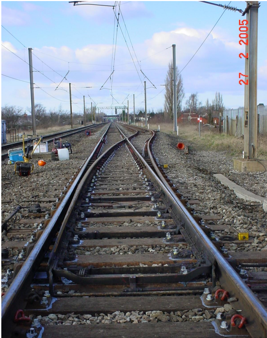
Figure 21: Completed high speed turnout Oxheys West Coast Main Line
