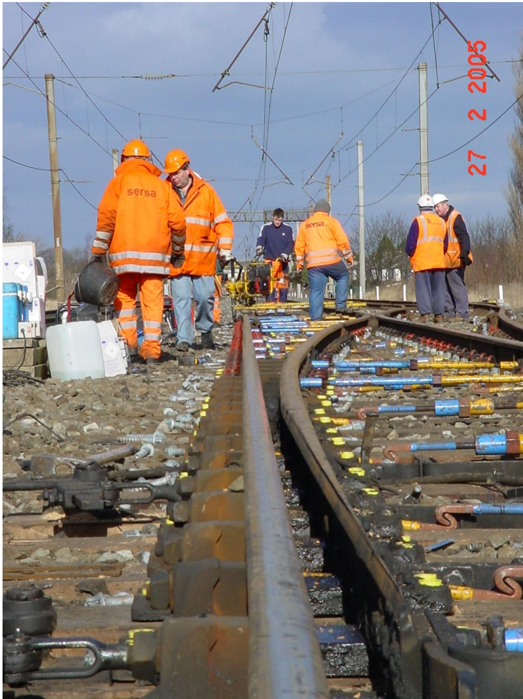
Figure 23: Sersa Second Life Timber Treatment System (courtesy Sersa-UK Ltd.)
