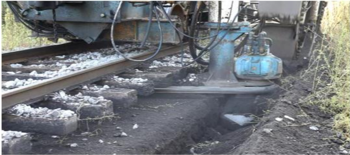
Figure 15: BBI Undercutter ballast and formation preparation machine (Source: bbinc.com)
