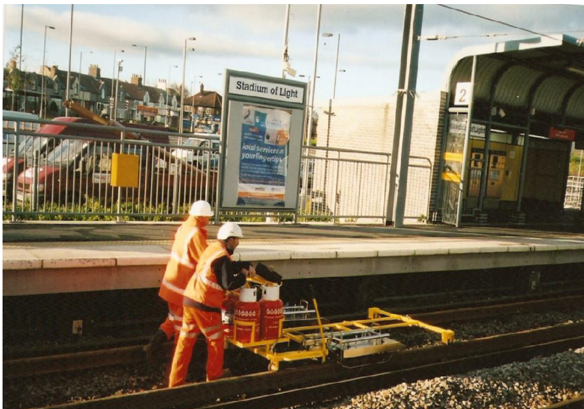
Figure 26: Sersa heater rail restressing System (courtesy Sersa-UK Ltd.)
