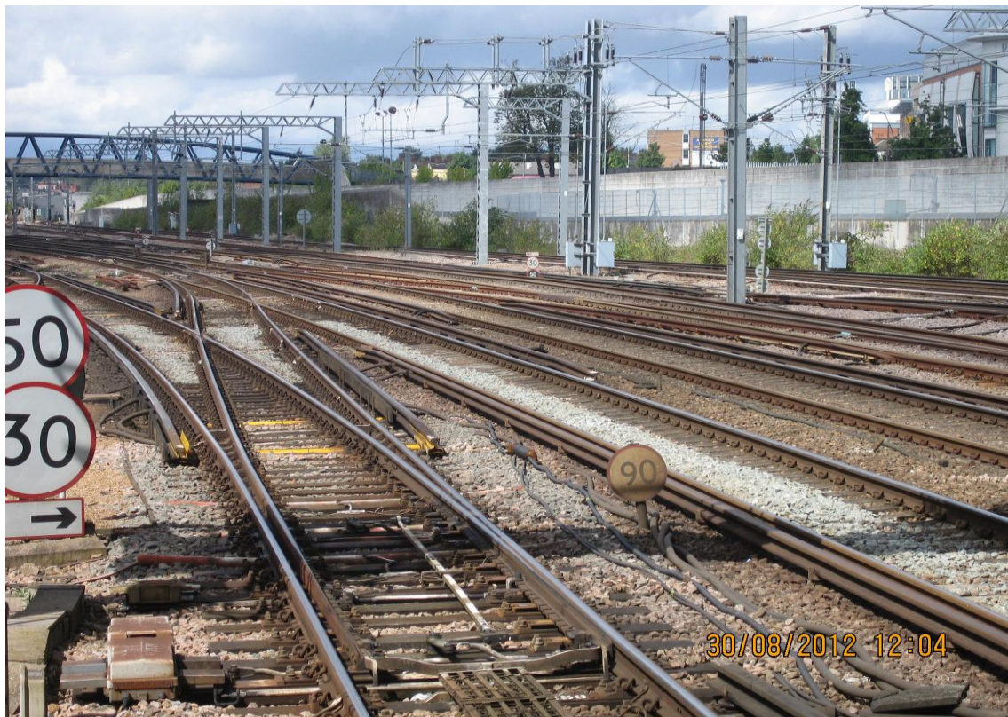
Figure 45: Completed Works at Ashford International Station (Source: author)
