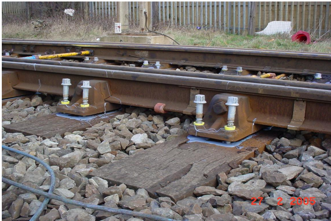
Figure 11: Second Life System in Progress Oxheys Preston UK (courtesy Sersa-UK Ltd.)
