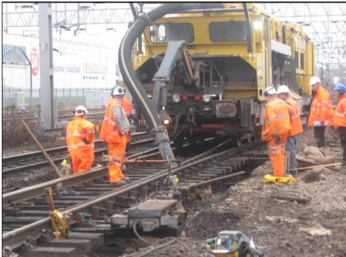
Figure 12: Railvac working at Stafford on West Coast Main Line 2007 (Source Sersa-UK)
