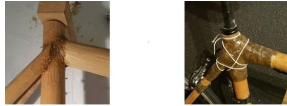
Figure 4. Making the connection and joints
