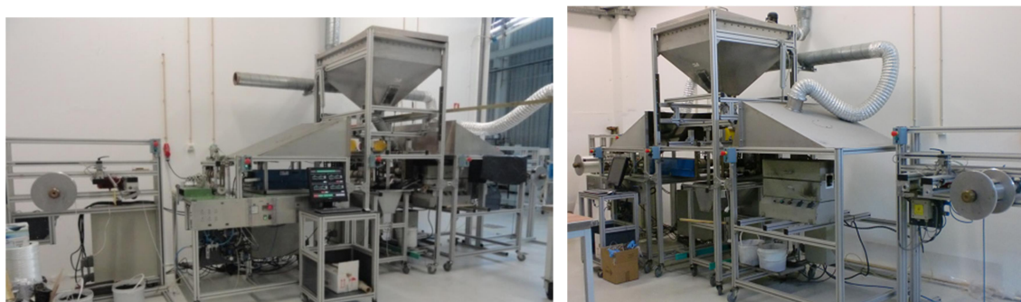
Figure 2.32 - Powder coating line setup
