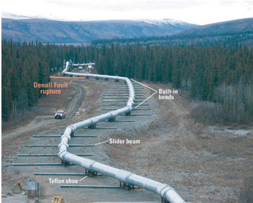
Fig. 10.8 Trans-Alaska Oil Pipeline and Denali Fault crossing (USGS 2003)
