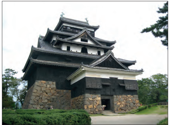
Fot. 11. Drewniany zamek w Matsue (fot. autor) Photo 11. Timber castle in Matsue (photo by author)
