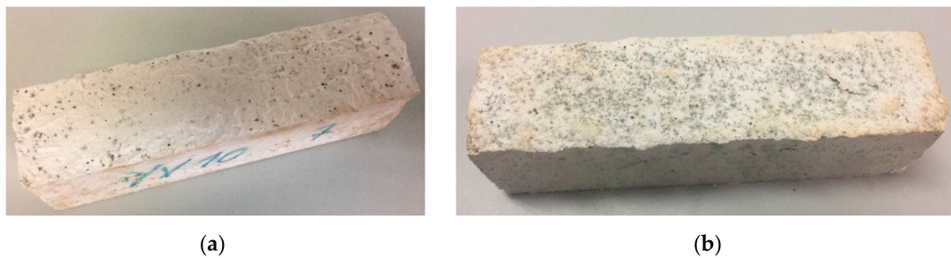
Figure 6. Small spots of mildew in wood shavings plasters after 15 wetting–drying cycles. (a) WS10; (b) WS20.
