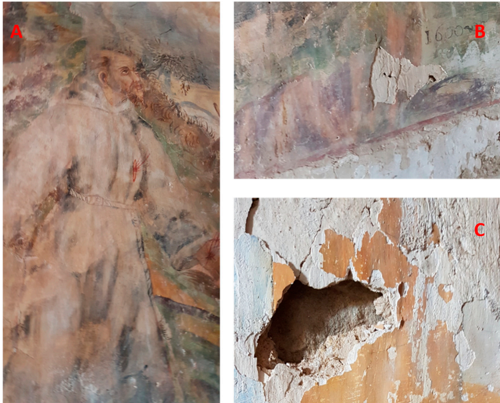
Figure 7. Details of the wall painting: (A) San Francis; (B) and (C) layer detachments.
