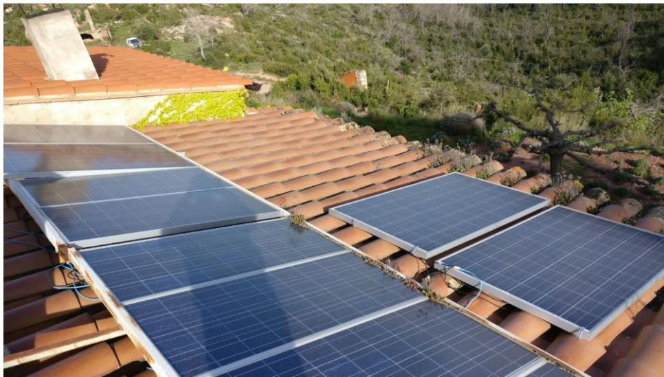
Figure 4.1 Solar Panel installation, on the roof of the house.
