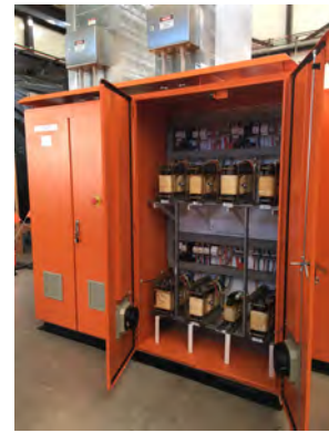
Fig. 12. Adjustable load bank (ALB).
