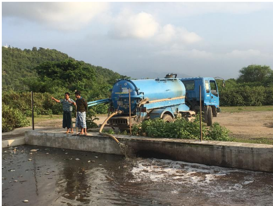
Figure 7. FS truck discharging into the oxidation pond. Source: J.Sanchez
