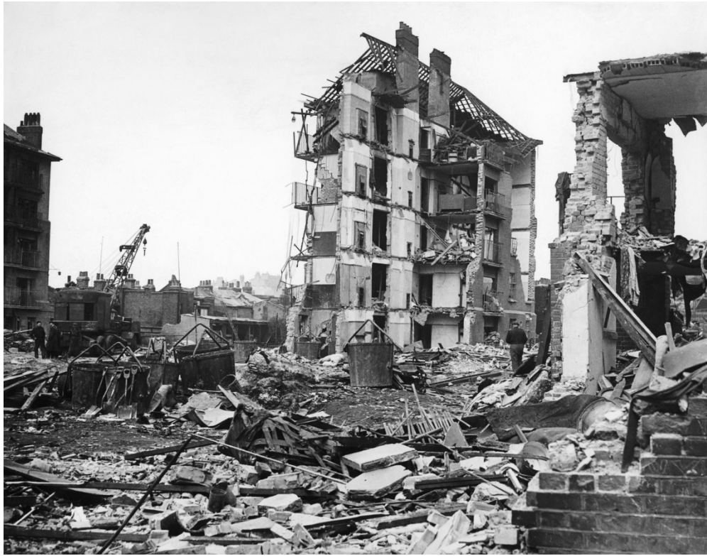
Figure 1. After-effects of a V-2 strike on Hughes Mansions, Vallance Road, London at 7.21 a.m. on March 27th, 1945, that killed 134 people. © IWM (HU 88803).
