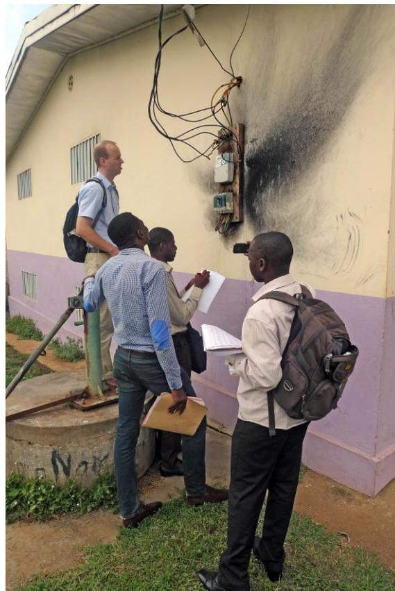
*Figure 2 : Inappropriate electrical wirings or unbalanced/overcharges phases are causing many fire in electrical installation like on the picture taken in one of the audited hospitals.*
