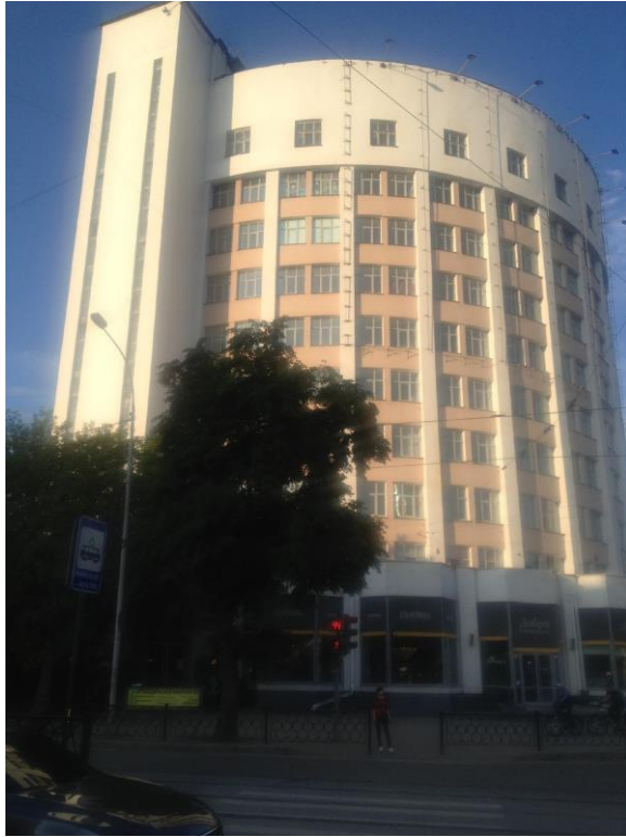
Figure 5.15. ‘Iset’ building, Chekist City, Yekaterinburg. (Photo by author)
