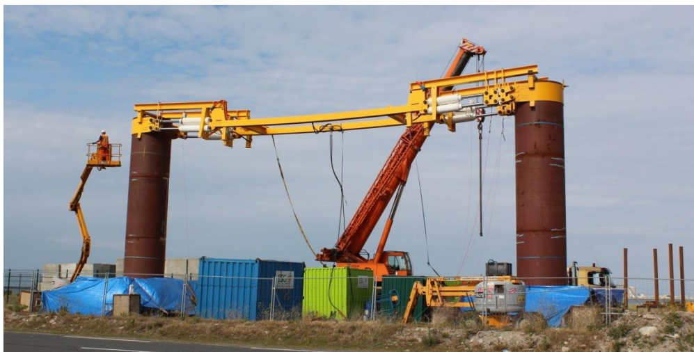
Figure 4: Photo of 2.0 m diameter pile tests at Dunkirk, France.
