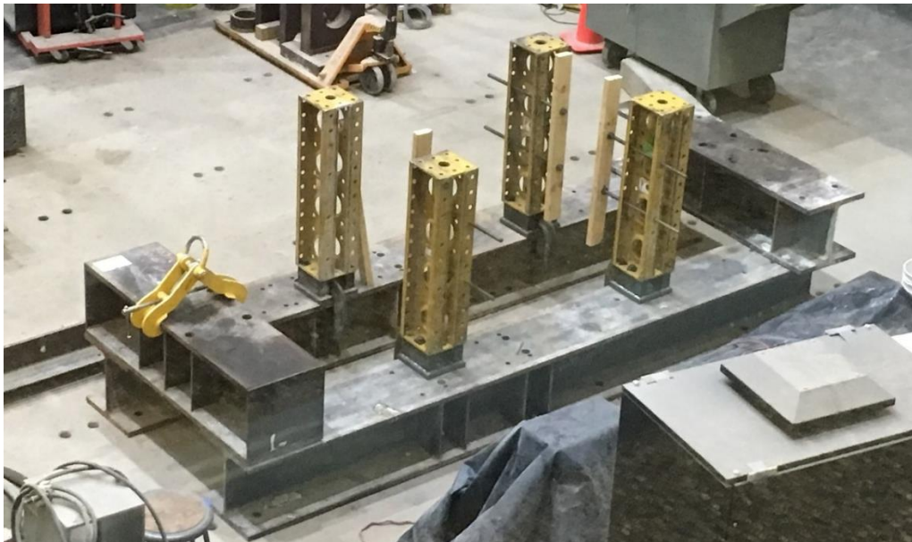
Figure 4.21: Bracing viewed from above
