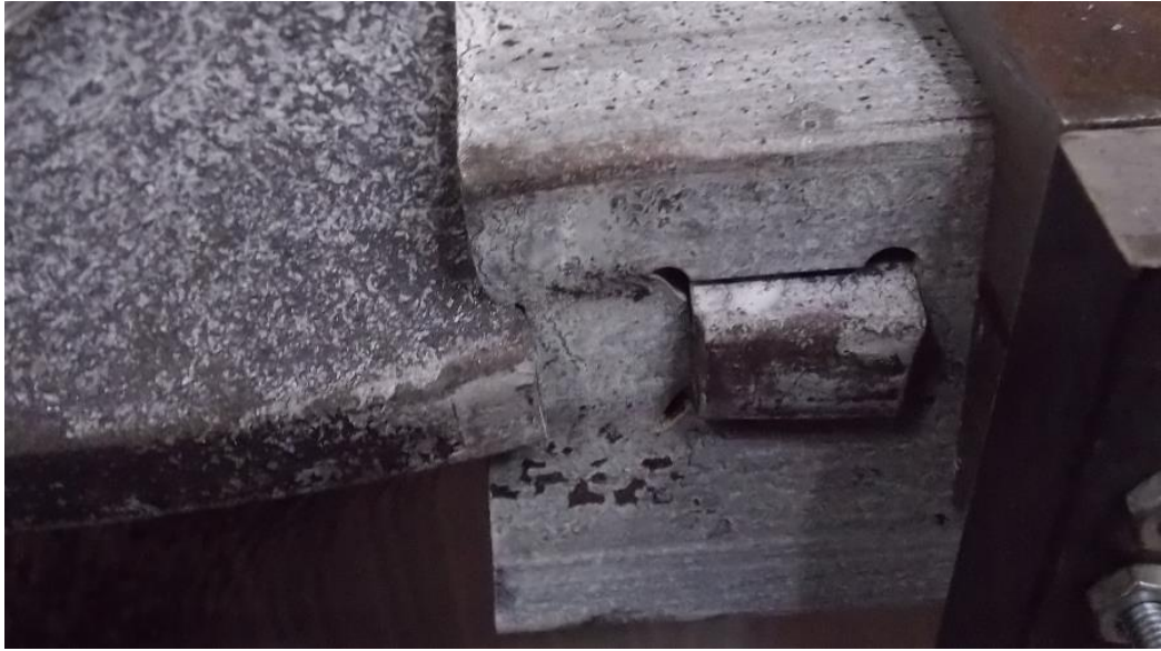
Figure 5.4.12: Deformed beam flange loading the angle at peak load
