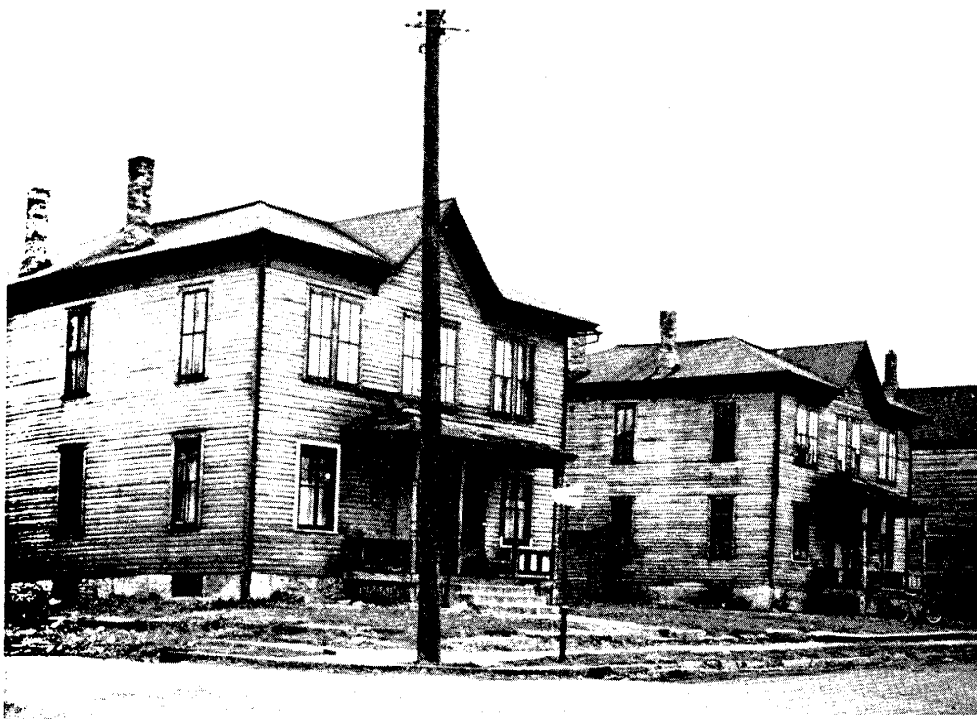
The Glenwood Homes site, mid-1950s.
