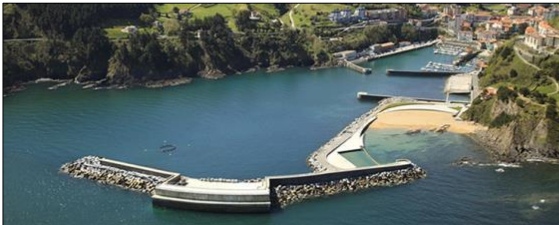
Figure 21. Mutriku Wave Power Plant project
