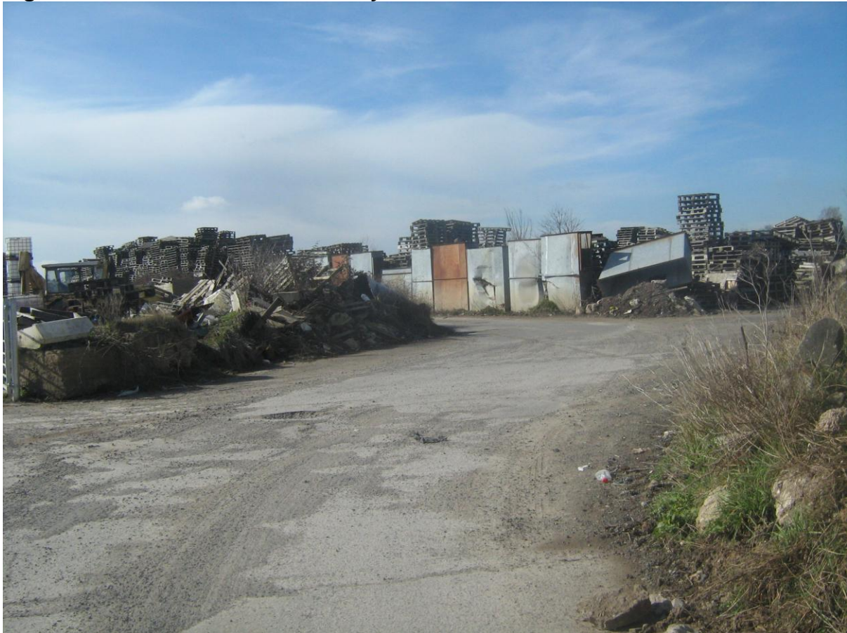
Figure 4.5.3 Entrance to Westonzoyland site
