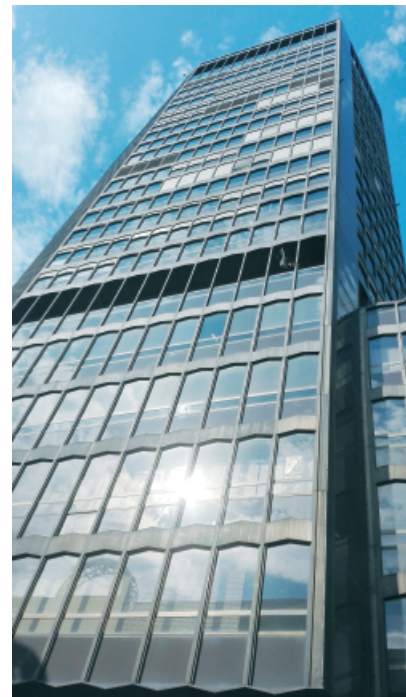
Figure 5. Belgrade Palace tower, detail of glass façade
