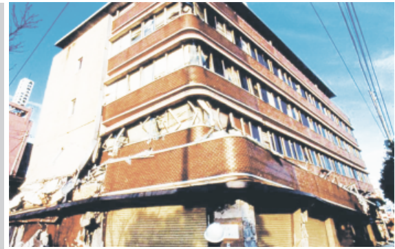
Figure 1. Torsional fracture due to arrangement of walls in the 1995 Kobe earthquake [13]
