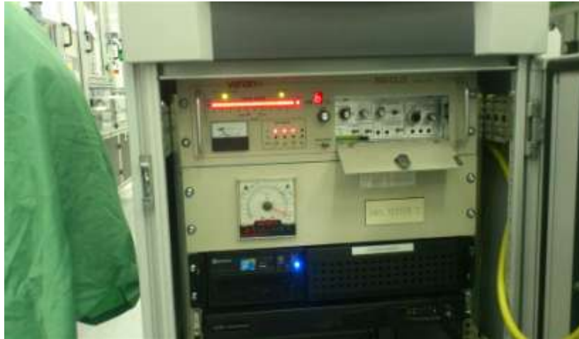
Figure 7. The helium leak detection device
