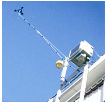
Figure 1. Local meteorological station on school building roof
