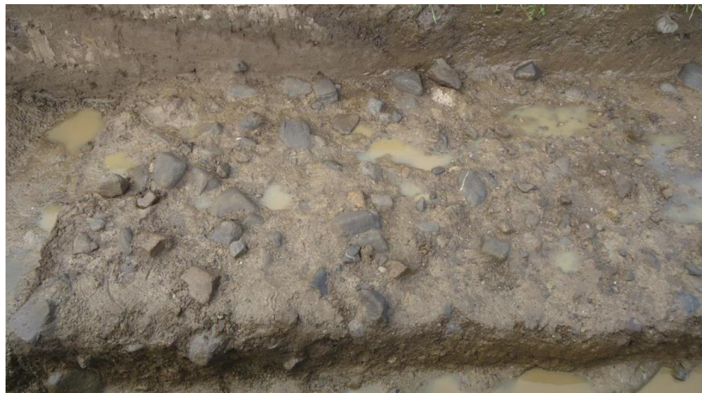
Figure 28: Roadway excavated in DS1, composed on limestone cobbles within a clayey soil matrix (Brady et al. 2017).
