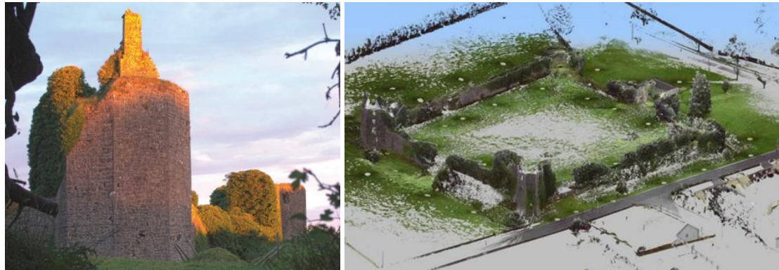
Figure 13: Northwest corner tower of Ballintober Castle (Brady et al. 2018) and laser scan of Ballintober Castle (Brady 2014).
