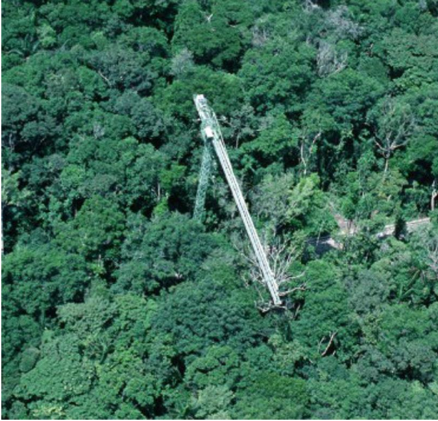
Figure 154. Canopy crane at Surumoni, Venezuela. Photo courtesy of Robbert Gradstein.
