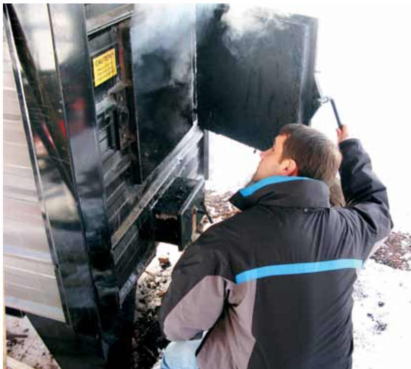
Team member Ben Stenske checking out the wood boiler
