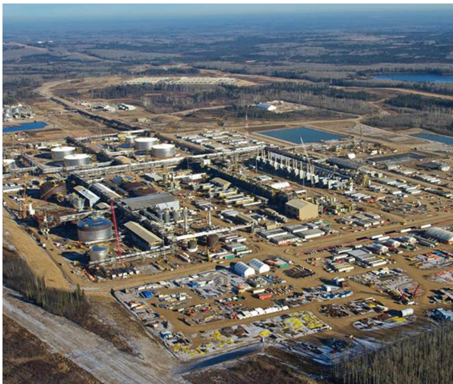
Conoco Phillips Oil Sands Surmont Operations Facility in Alberta, Canada
