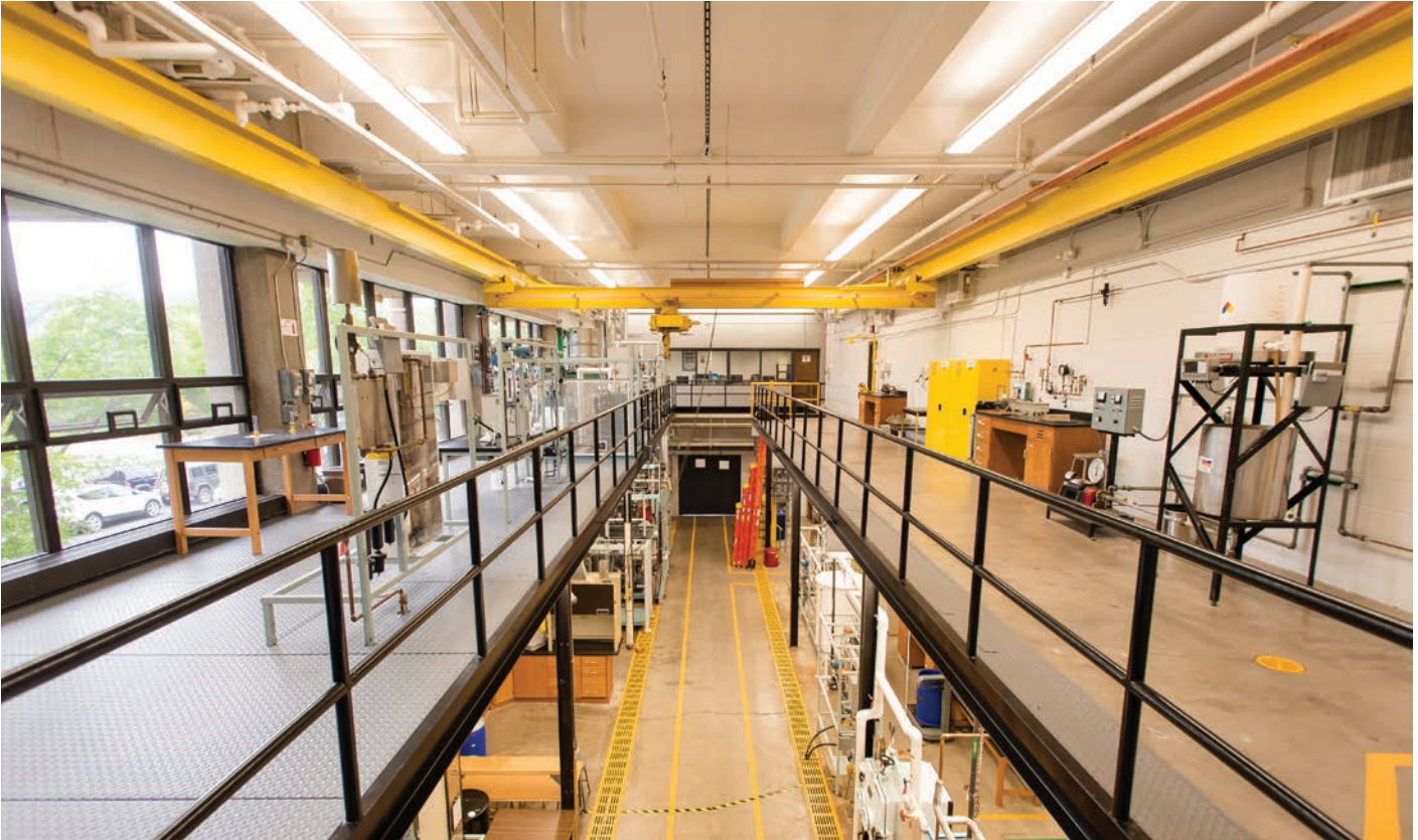
Panoramic view of the first and basement floors of the UO Lab North Wing
