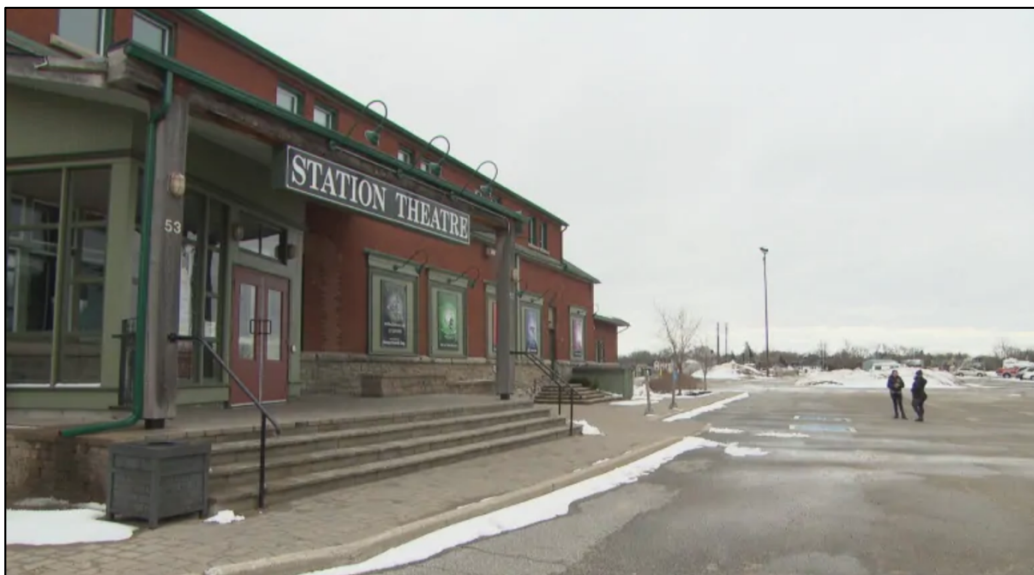
Figure 51: Smiths Falls' former railway station – now a theatre. Courtesy of Skura 2018.
