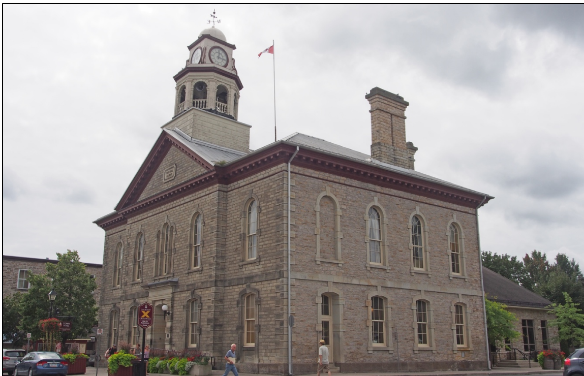
Figure 12: Perth’s Town Hall. Courtesy of Raué 2018.
