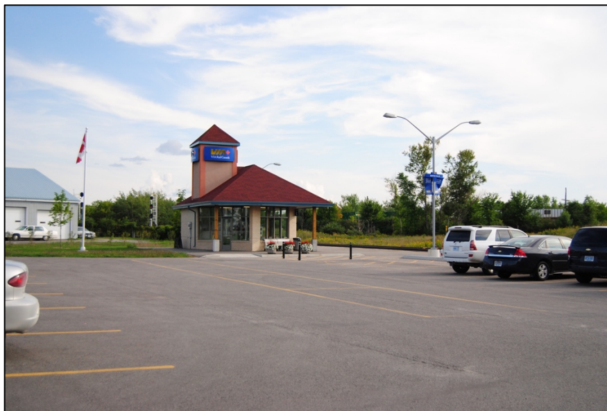
Figure 52: Smiths Falls' current VIA station. Courtesy of Canadian Public Transit Discussion Board Wiki 2013.
