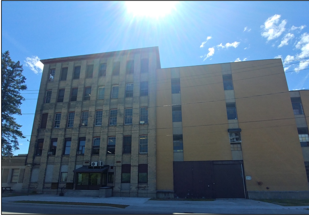
Figure 55: The Perth Soap factory building, now Shandex Personal Care Manufacturing Inc. Photo taken by author.
