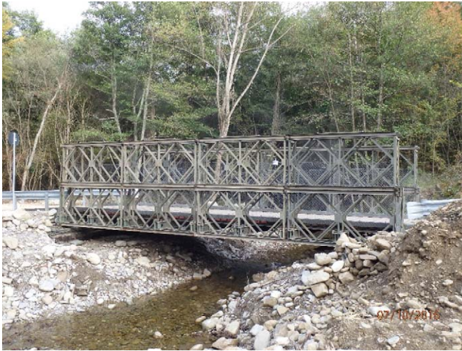
Figure 13. Temporary bridge near Ponte Rosa .
