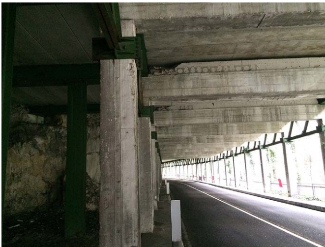
Figure 10. Overview of the composite steel-RC rockfall protection tunnel near Norcia.
